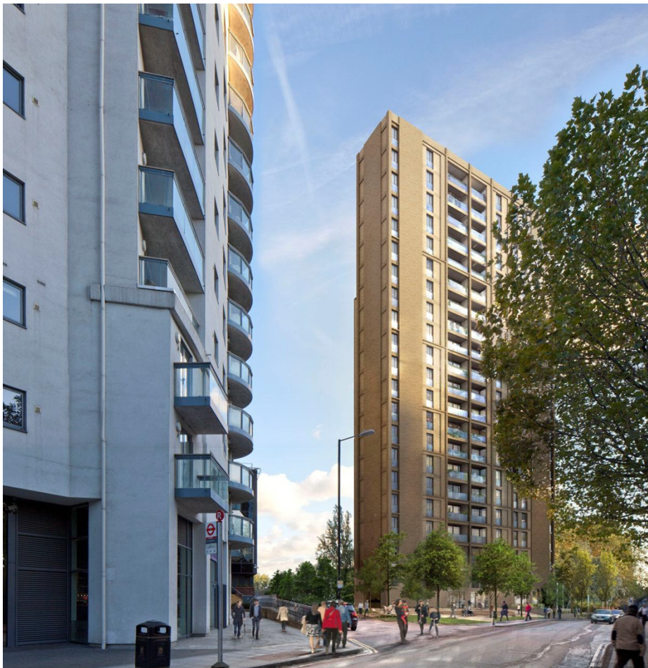
Figure 4: CGI of west elevation with No 3 (City Tower) to the left
